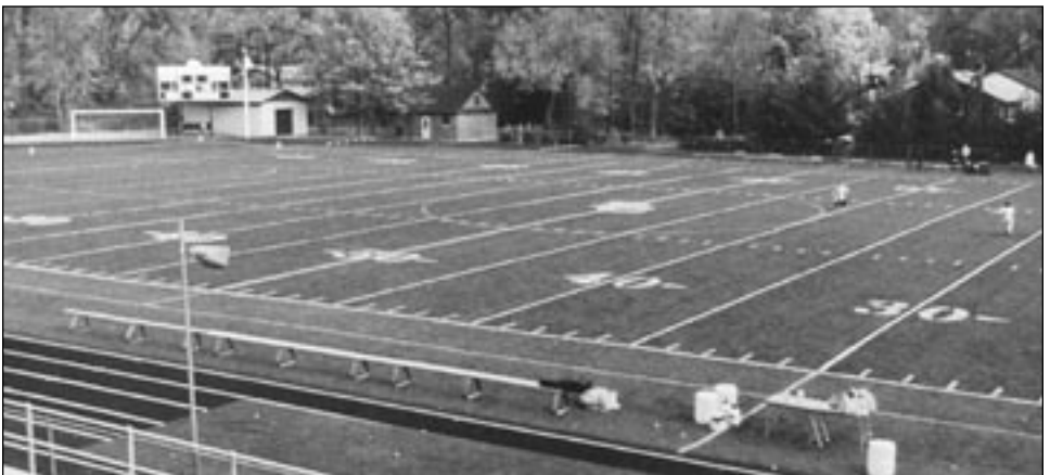
FieldTurf™ was installed on the BC football field in 1998.
